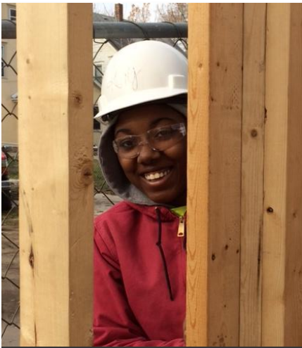
Keiona rehabbing a home in North Minneapolis.
